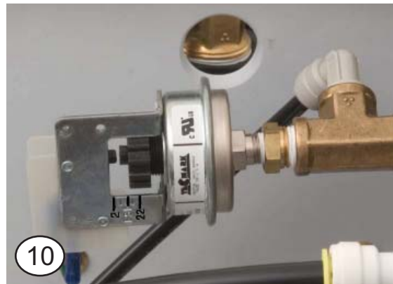
Low Pressure Switch shown set at 10 psi and is un-pressurized
