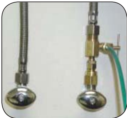
INSTALL ON COLD WATER LINE
